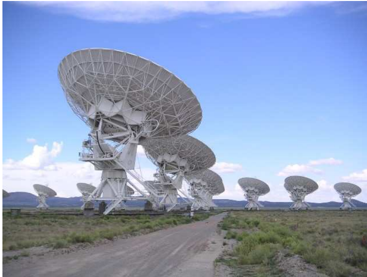
Figure 13. VLA array in New Mexico has 27 antennas each 25 meters in diameter. The antennas can be moved up to a maximum baseline of 22 miles
